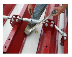
Panels are positioned, aligned, stacked, and secured to appropriate heights.
