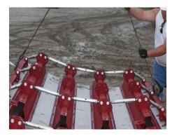
Tie Rails, scaffold brackets and braces are attached and lifted onto prepared foundations.
