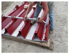
CIRCA-FLEX arrives flat and simply turning the turnbuckles changes the radius.
